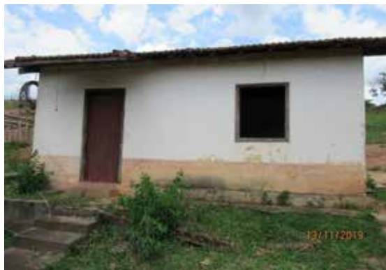
Fachada principal - Vista
